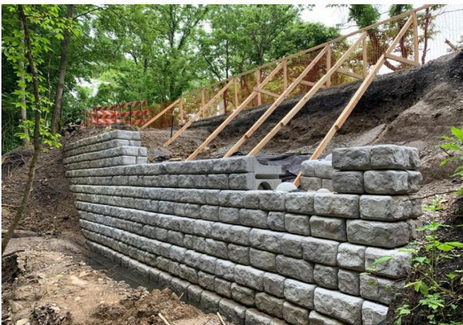
Retaining wall seen from below.
