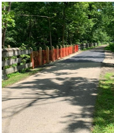
Trail above the retaining wall.
